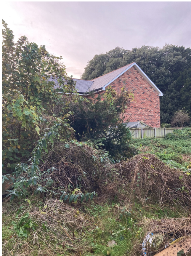
Figure 8: View looking west from within the site, towards No. 53 Church Path
